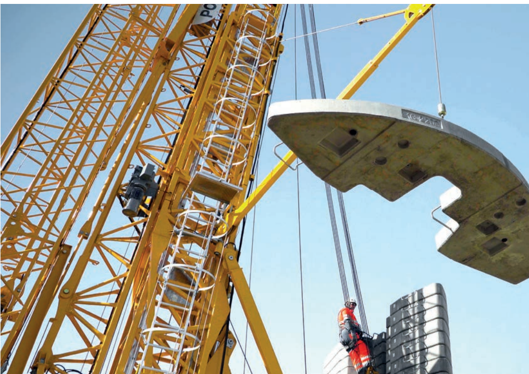
Hydraulic ballasting derrick specific for Igo T 99
